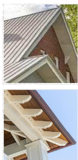
EXPOSED EAVES AND SHAPED RAFTER TAILS (2 FT OVERHANG & GREATER)
